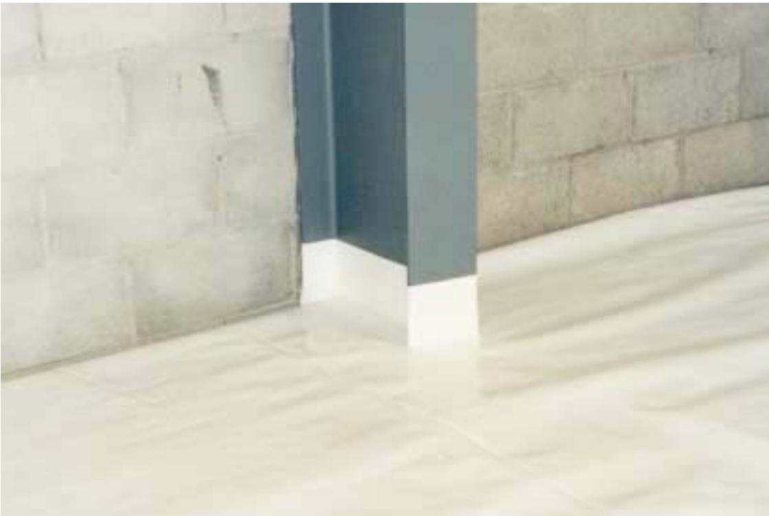
**Fig 3: Detail showing structural steel stanchion with penetration seal**
