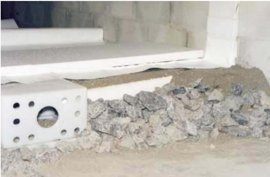
**Fig 5: Section through a sub-floor showing the installation of a radon collection sump with proprietary white vent pipe system**
