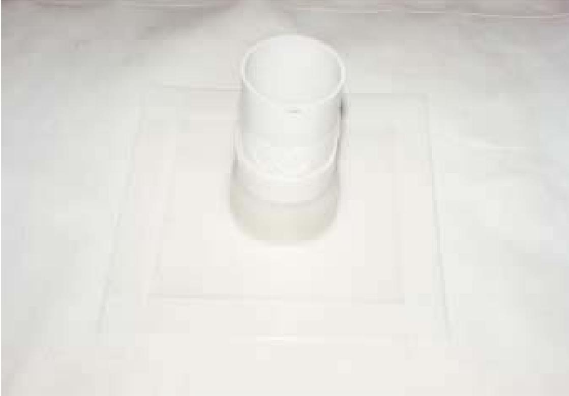
**Fig 2: Figure showing Top-Hat with Polyseal strips**
