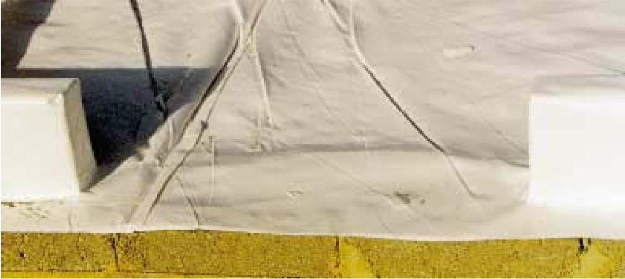
**Fig 1A: Factory sealed fusion weld joint and wrap around radon protection detail on rising wall at external door opening**
